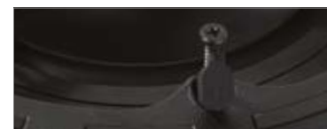
Stainless steel fixing screws with Neoprene covers
